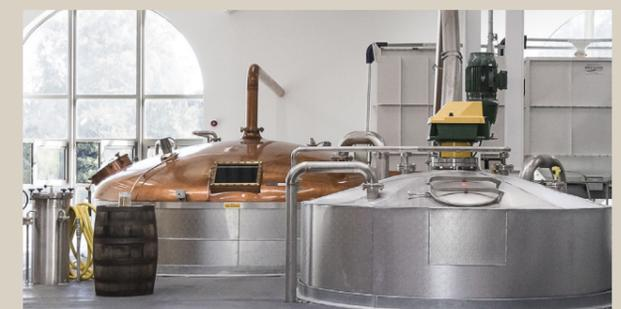
Powerscourt Distillery utilises 100% renewable biogas to make their whiskey and then harnesses the heat from the mashing process using heat exchangers to power the underfloor heating for the Visitor Centre.
